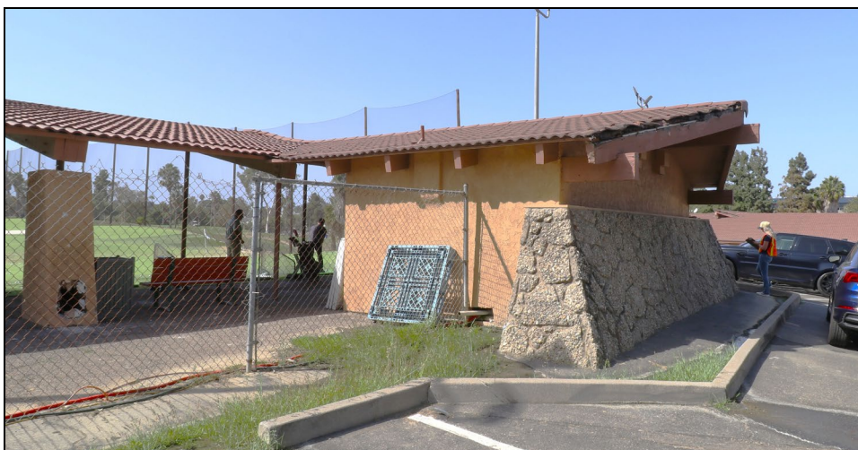
Driving range shack and canopy, view west (10/25/24). Note the stucco-wrapped pole (far left), extended gable peak (far right), and concrete and pebble stone accent wall.
